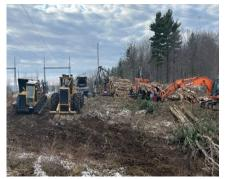
**Site Preparation:** The first phase of site preparation and construction is tree & brush clearing. There will be ~14k LF of non-contiguous new tree cutting (ranging in width from 0 to ~60 ft) along the ~111k LF project length.
